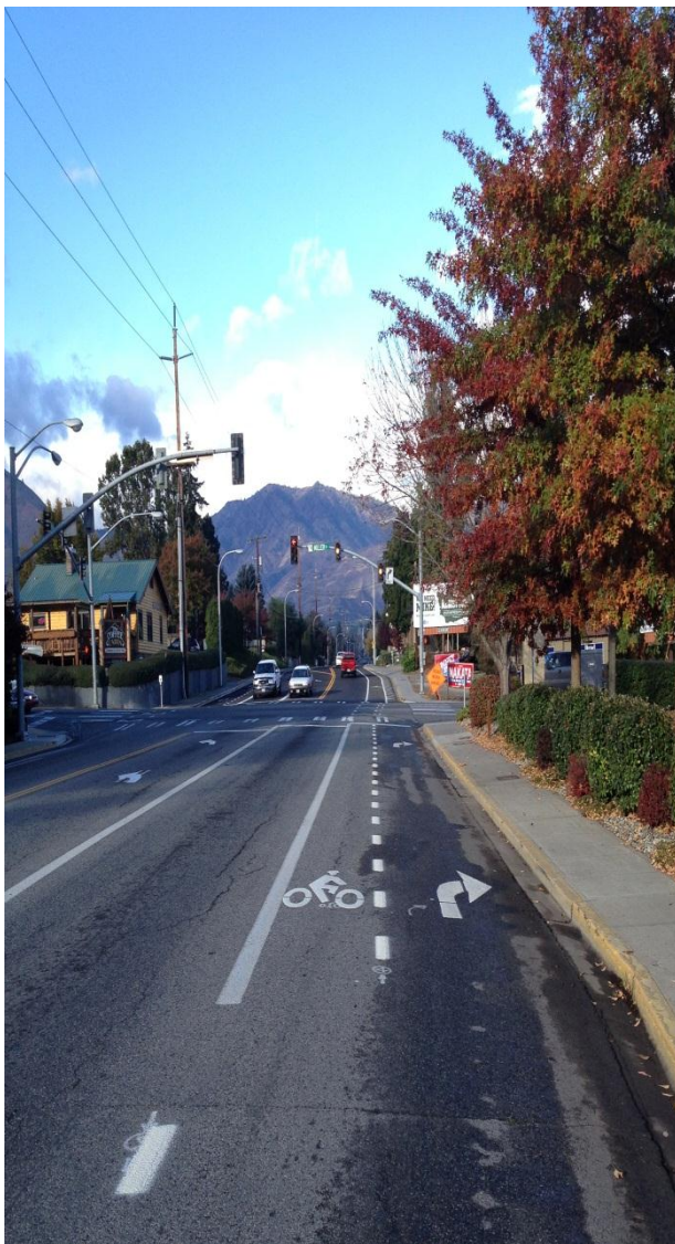
PHOTO 8-SHARED RIGHT TURN LANE @ 5TH AND MILLER INTERSECTION
